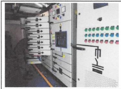
Picture 3 Main Distribution Board preventive maintenance.
