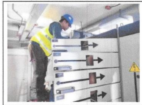
Picture 3 Main Distribution Board preventive maintenance.
